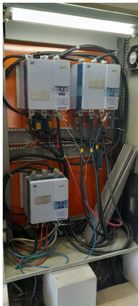
Painel Elétrico Geral / Painel com chaves Soft Starts
