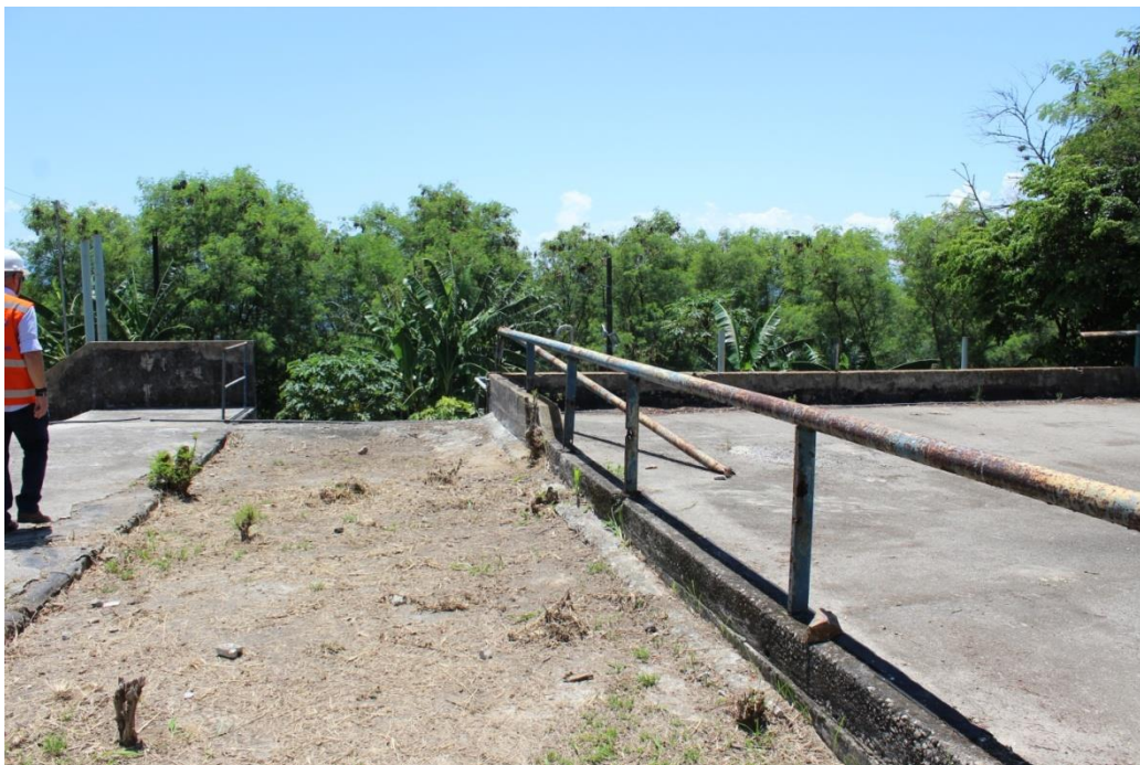
Grade Deteriorada
